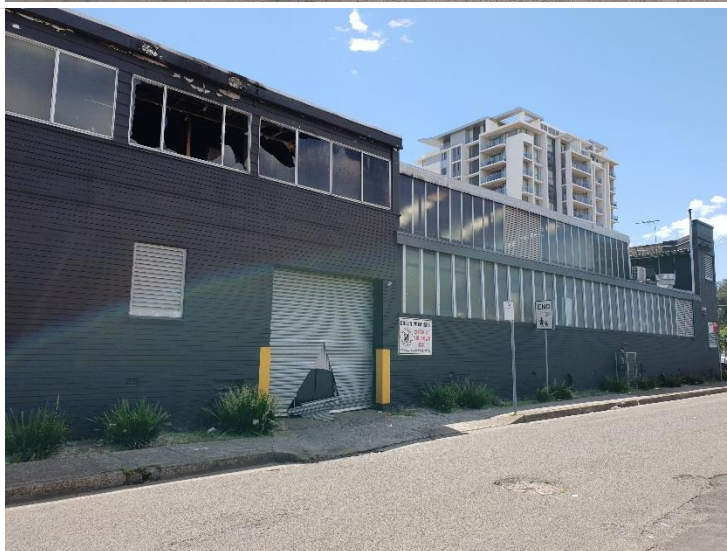
Photograph 2: View of the south-eastern section of the site. Note the charred appearance of the upper section of part of one of the buildings.
